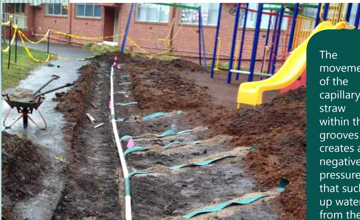
The movement of the capillary straw within the grooves creates a negative pressure that sucks up water from the soil.
