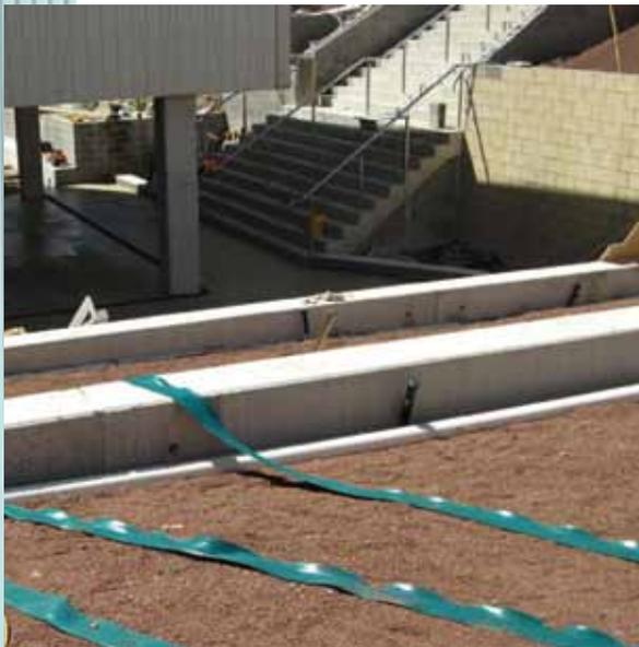
Capiphon™ drains best when the belt is in direct contact with the soil, obviating the need for a gravel transition layer.
