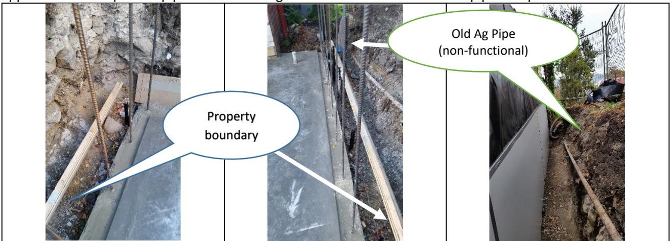
The area behind the new wall was excavated below the slab and a bed of FCR compacted to a level below the slab.
