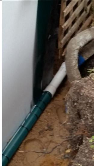
The Capiphon Pipe plugs into the special connector to join the stormwater system.
