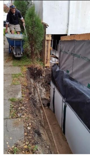
Covering the Capiphon Pipe with coarse sand before backfilling the trench.
