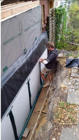
Strips of Capiphon Belt inserted into the Capiphon Pipe, and taped to the core flute sheets.
