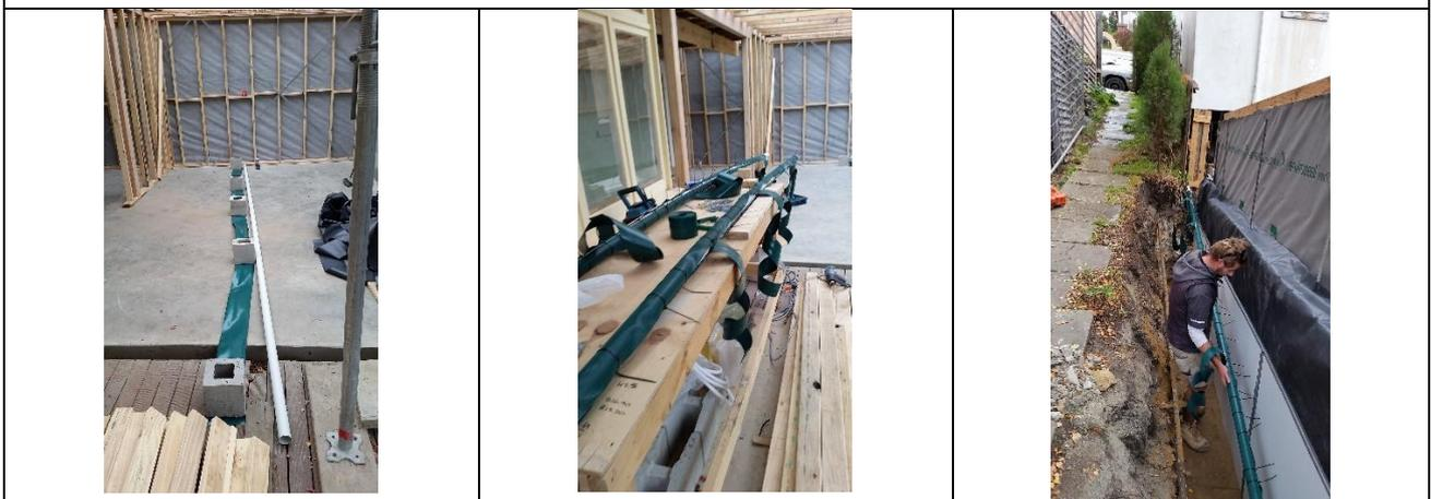
Capiphon Pipe being fabricated on site before being laid on a thin layer of coarse sand.
