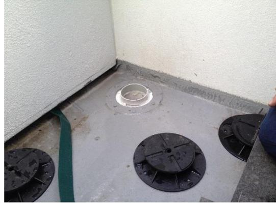
The connector is made from PVC pipe with a slot cut into it to take 5cm wide Capiphon belt. The connector was sealed into the drain pipe and the belt inserted into the slot and sealed above and at the sides with silicone sealant.
