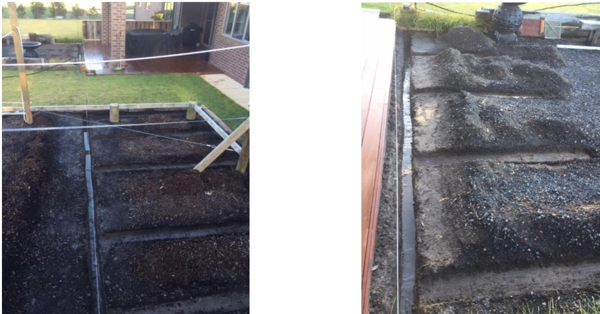
**PICTURES# 5&6:** Images showing fabrication of collection pipe with Capiphon and insertion of Capiphon belt into the collection pipe.
