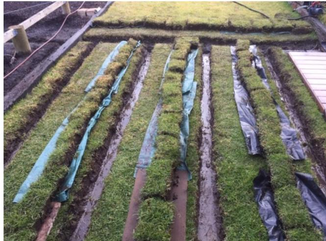
**PICTURE# 8:** Image showing placement of Capiphon belt and Capiphon collection pipe in soft-fall/playground area
