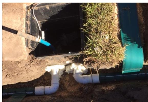
**PICTURE# 10:** Image showing water draining from Capiphon system into submersed pit. After 30 minutes of rain, water began to drain into pit. Three hours following rain, water was still being syphoned through the Capiphon system and being dispersed into the drainage pit.
